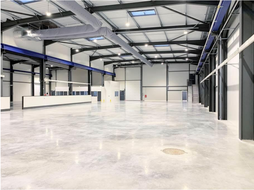
Fig. 2: Production hall at the new location (Photo: WITTMANN BATTENFELD France)
