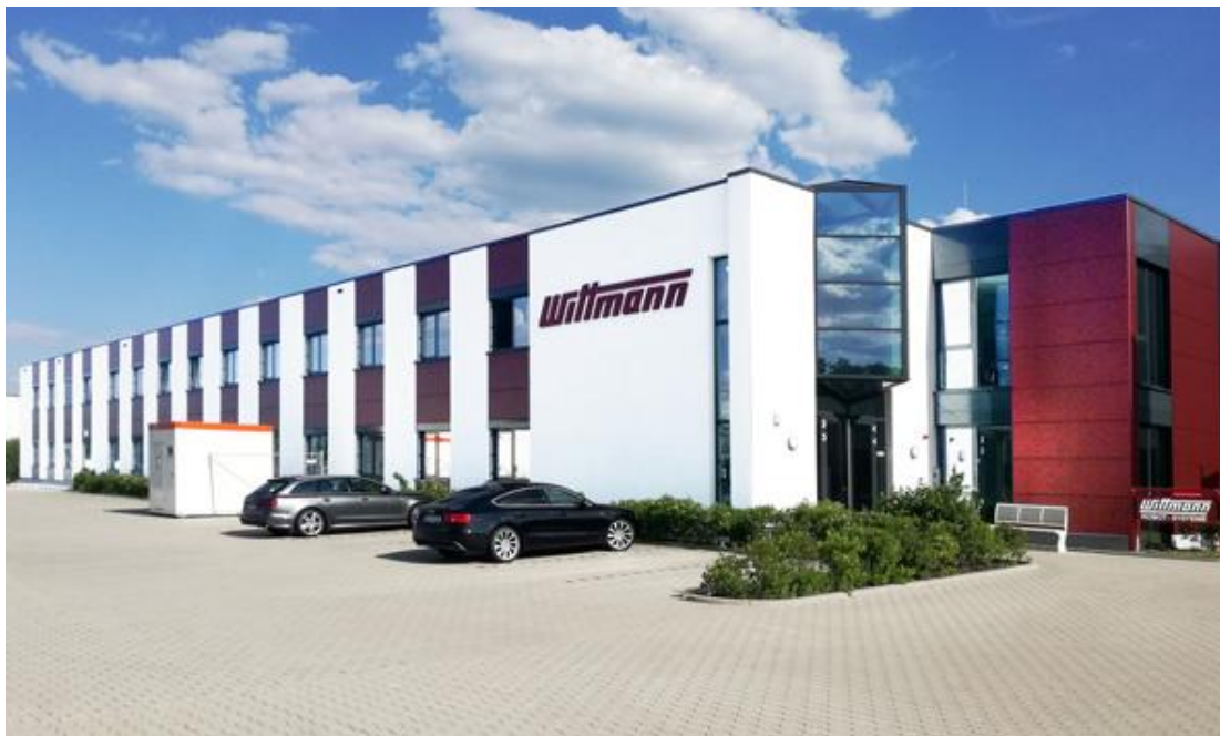
Shown on the left in this picture: the office tract of WITTMANN Robot Systeme in Nuremberg, extended by a total of 17 m. The remaining work on the outdoor areas will be completed by the end of June.
